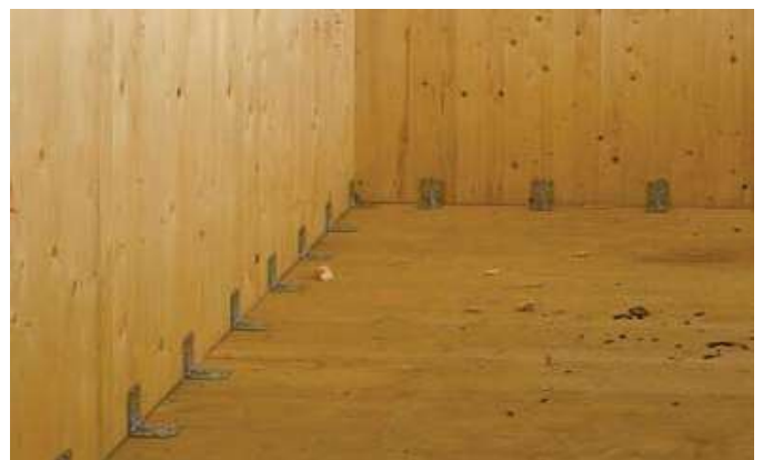
Figure 8. CLT wall floor connection – Murray Grove [13].
