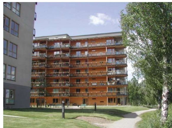
Figure 11. Limnologen apartment buildings, Sweden.
