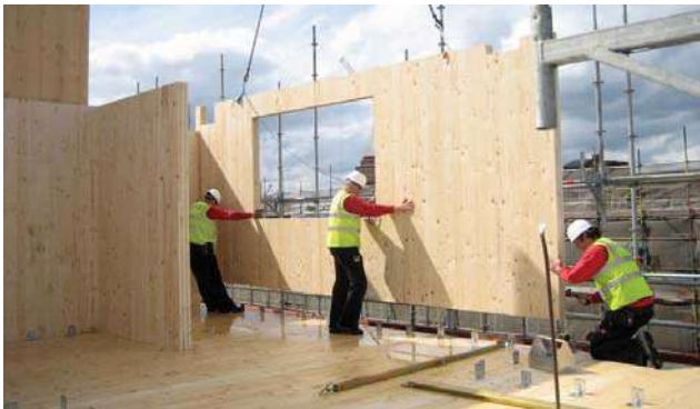
Figure 3. Platform construction – Murray Grove [13].
