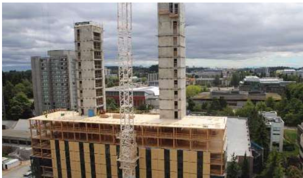
Figure 17. UBC student residence under construction
