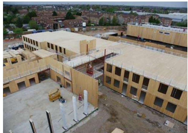
Figure 14. Mayfield school – construction phase [28].
