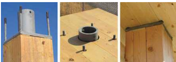
Figure 18. Floor column connector [29].
