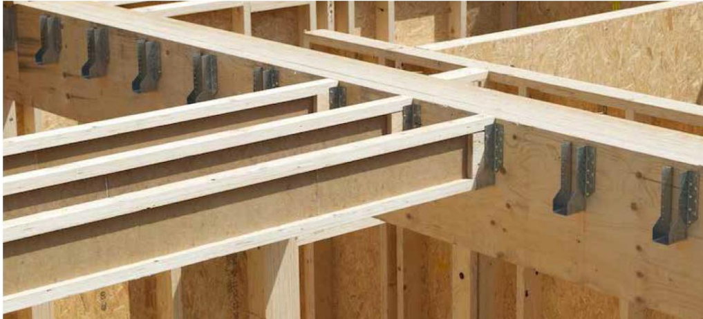
Figure 3.2 I-joist structural elements on metal joist hangers (photo: Steico 2020)
