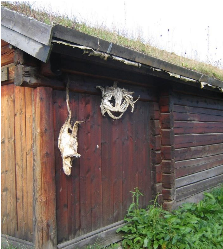
Figure 3.5 Traditional construction in Norway, a combination of post-and-plank in the front area, and log construction in the back area (Photo: E. Shotton)
