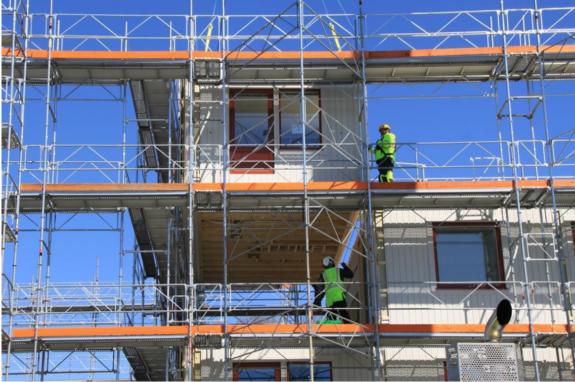
Figure 3.10 Assembly of multi-storey building made of volumes (Courtesy of Derome AB)
