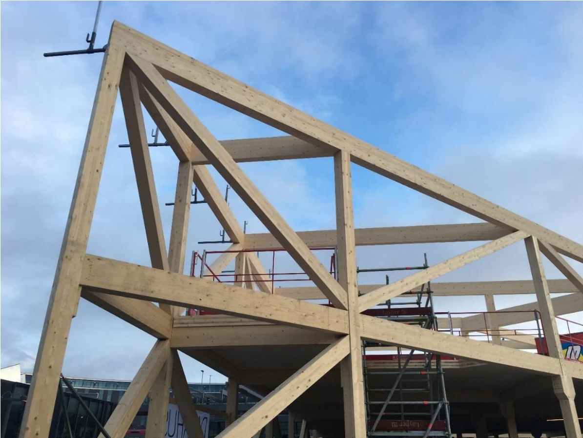
Figure 3.3 Post and beam frame (photo: D. Honfi)
