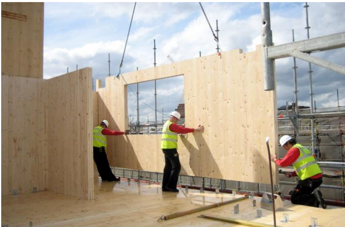
Figure 3.6 CLT Wall panels craned into position on construction site (Strongtie 2019)
