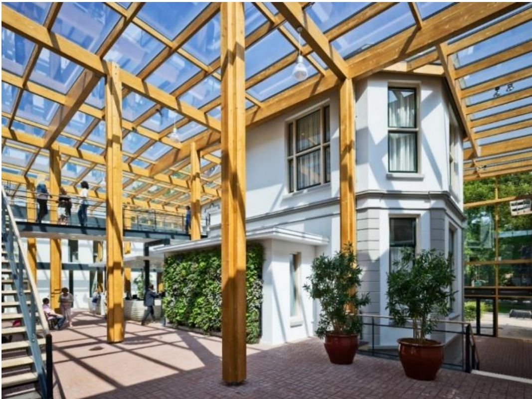
Figure 3.29 Brummen Town Hall, the Netherlands. Wooden structure planned for reuse (courtesy of Petra Applhof)
