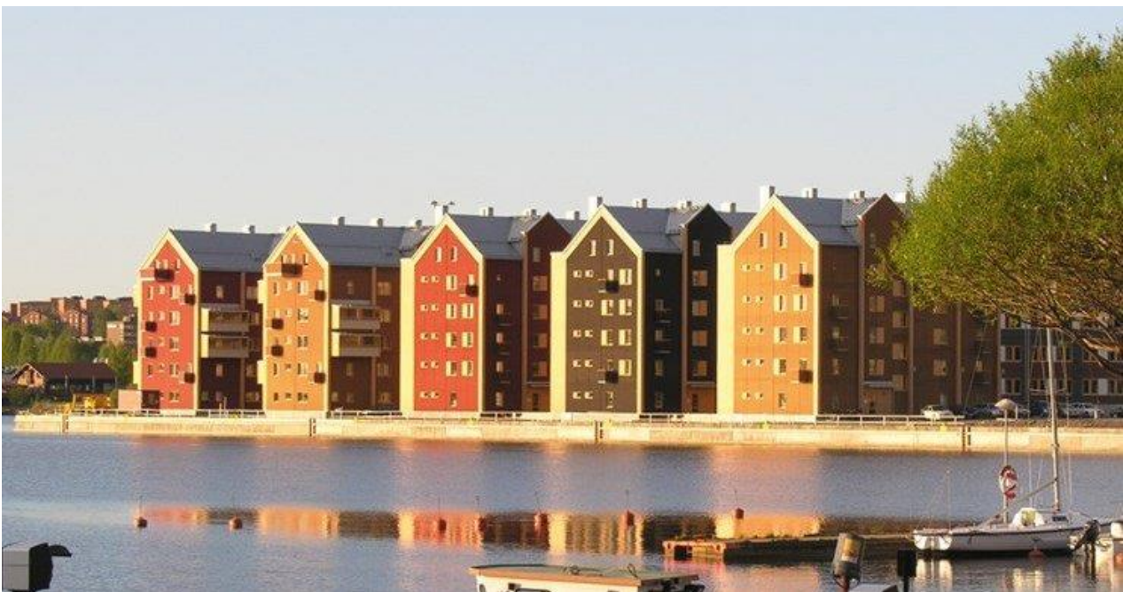
Figure 3.12 Inner harbour in Sundsvall, Sweden, year 2004. Five apartment blocks, from right to left: three blocks with a structural frame made from CLT, and two blocks with a light-frame building system. The wooden façade is of glulam cladding. Photographer: Per Bergkvist (Swedish Wood 2020)
