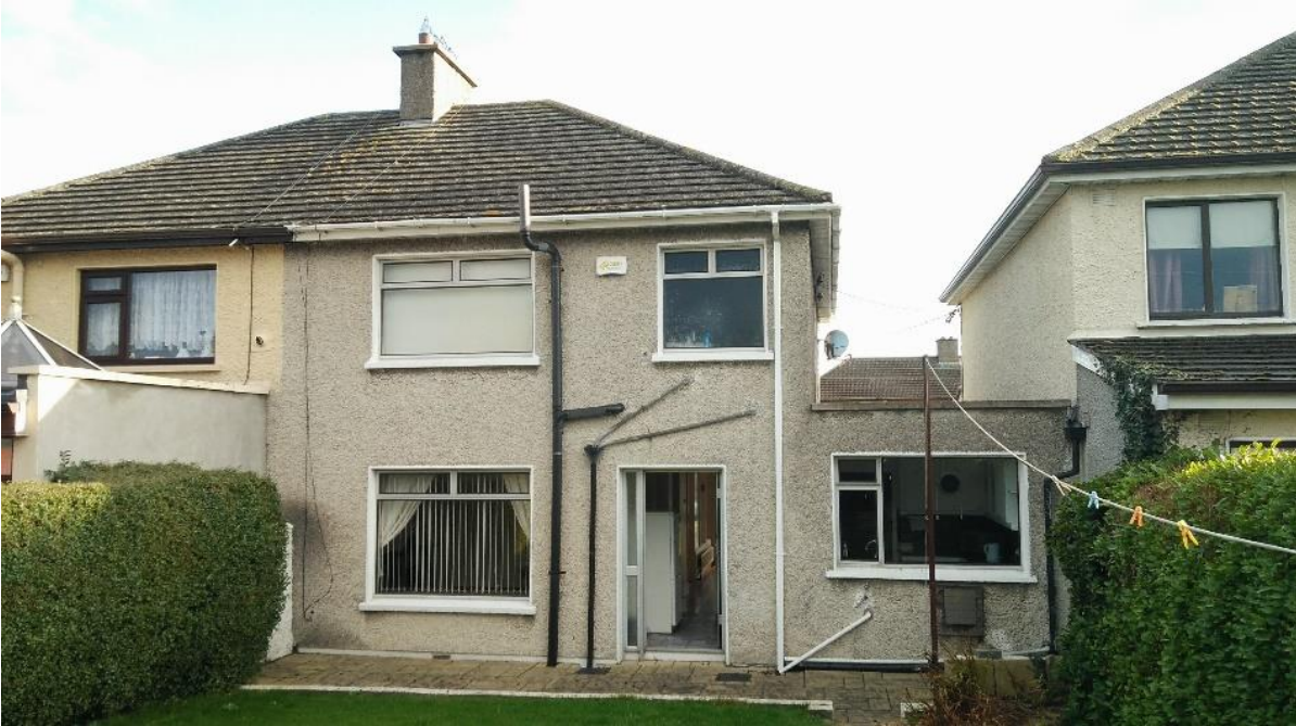
Figure 3.19 Conventional mid-20 th century load-bearing masonry house in Ireland (Photo: SJ Walsh)
