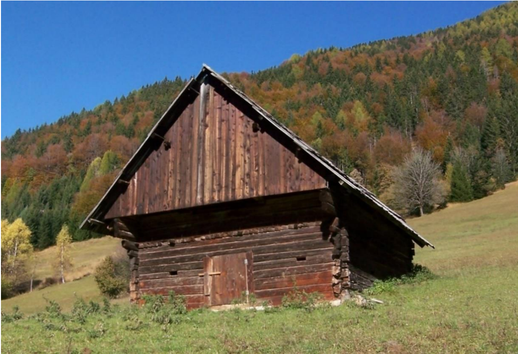
Figure 3.23 Old traditional wooden hut with shingles made of larch, in Kranjska Gora (Photo: Žiga Krofl)
