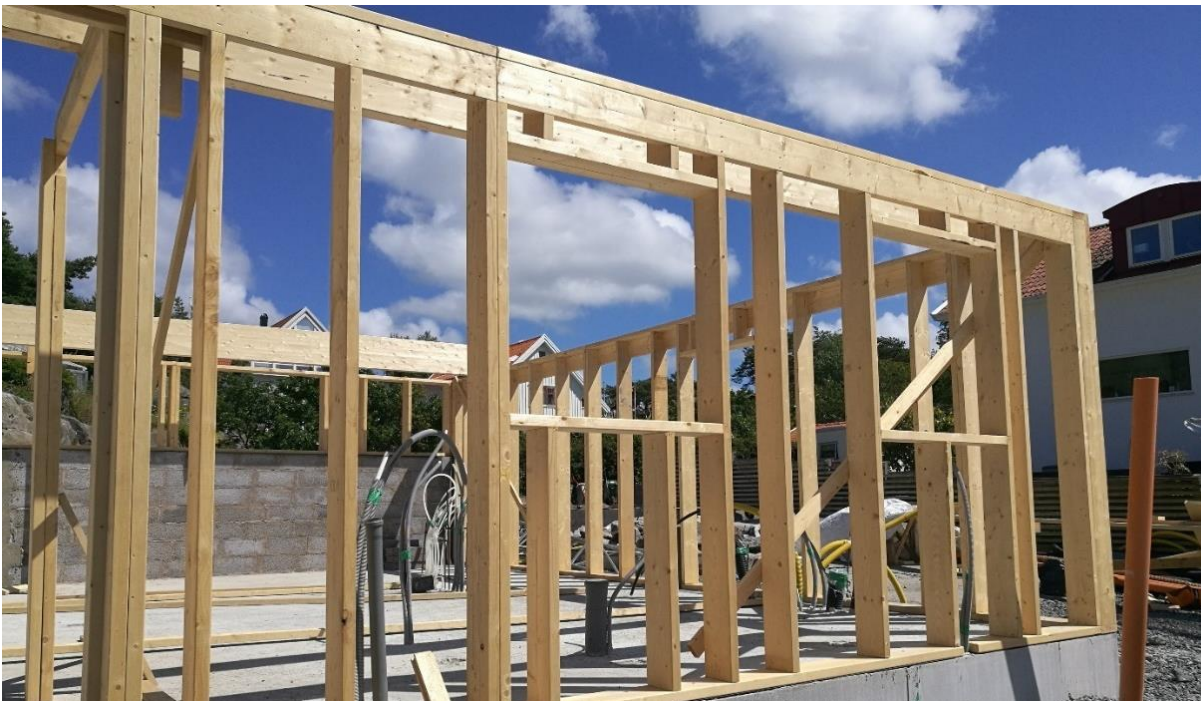
Figure 3.1 Example of onsite light frame family house (photo: D. Honfi)
