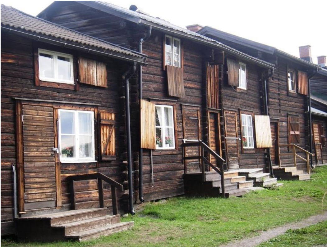
Figure 3.4 Traditional log construction from year 1830, "Bonnstan", Skellefteå, Sweden (Photo: Karin Sandberg)
