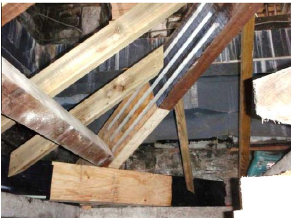
Fig. 28. Hip rafter repair [18].
