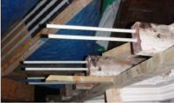
Fig. 20. GFRP rods inserted in ends of propped beams [18].
