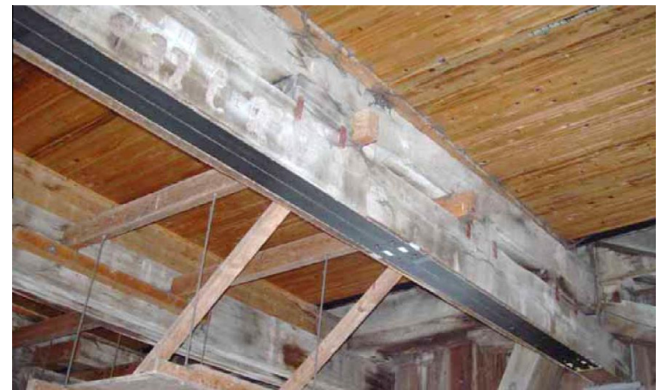
Fig. 30. Long-term monitoring of Sins Bridge, [57].
